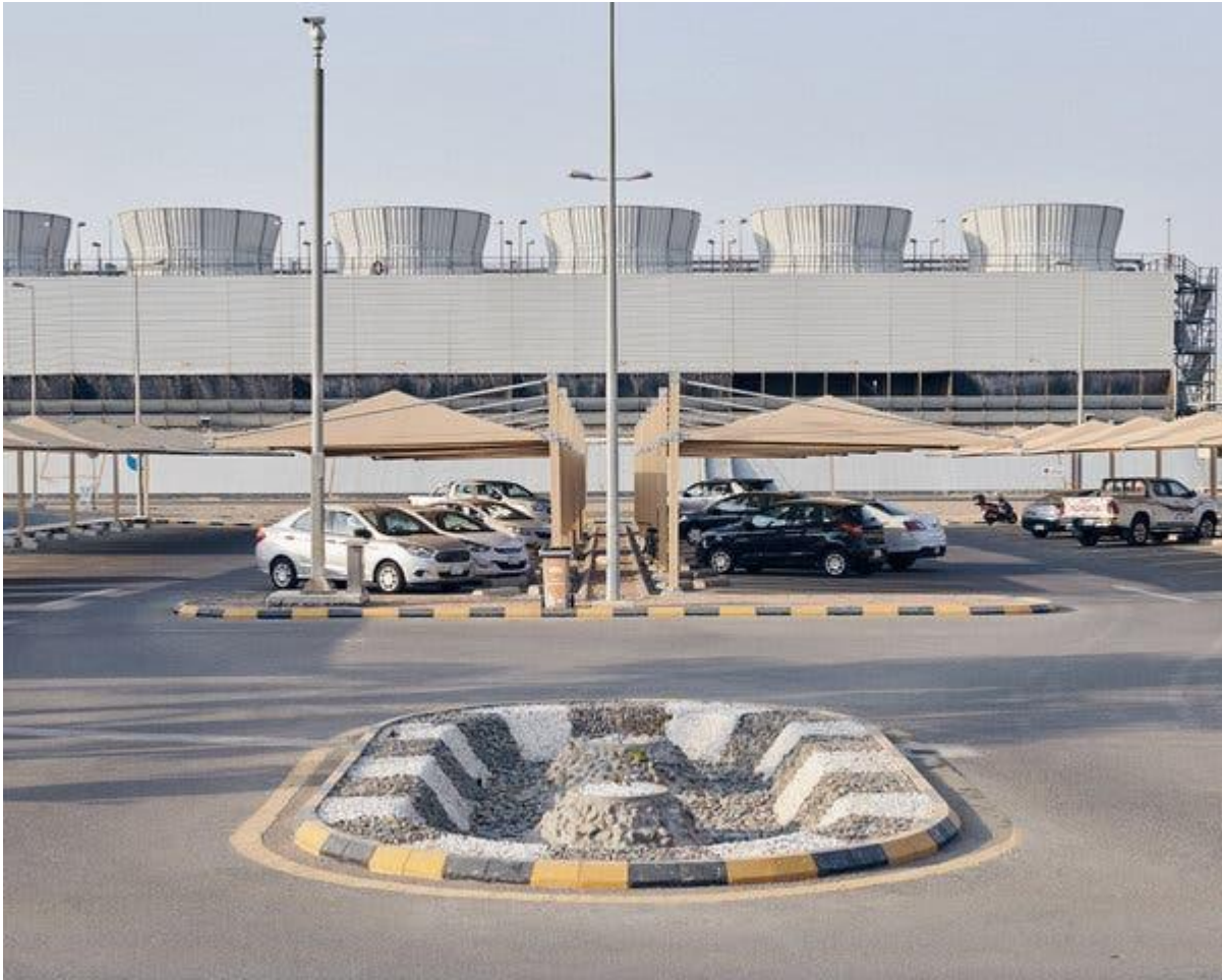
The Kaust desalination plant's parking lot. Cooling towers in the back, too, use desalinated water.
