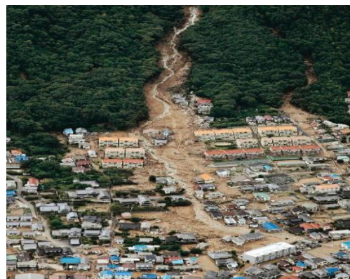
Landslide in Hiroshima prefecture
